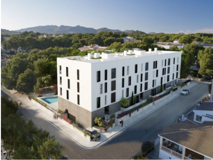
View to the building
